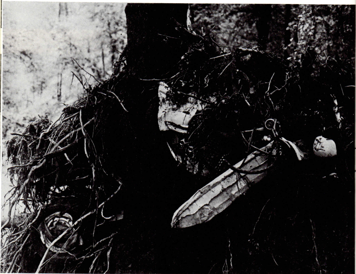
Flood debris along Tonto Creek near Kohl's Ranch. (Courtesy Ed Wiggins, The Mesa Tribune , Mesa, Ariz.)
